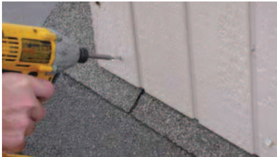
Secure chimney to roof using two (2) 2 1/2" screws along base of chimney on both sides.
