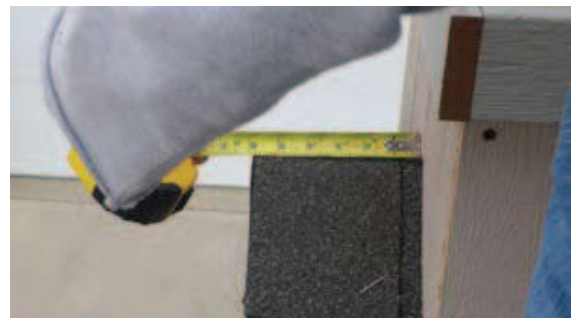
Carefully lift chimney to the roof. Measure inward 6" from end of roof and set chimney in place.
