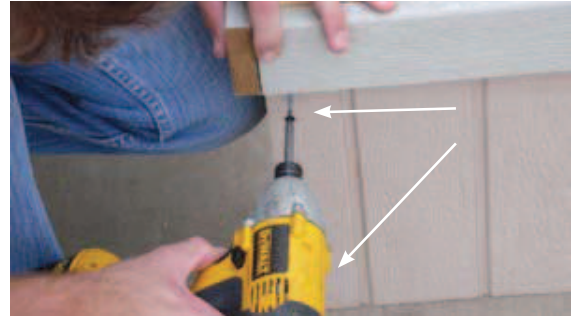
Secure corners of chimney using two (2) 1 1/4" black headed screws per side.
